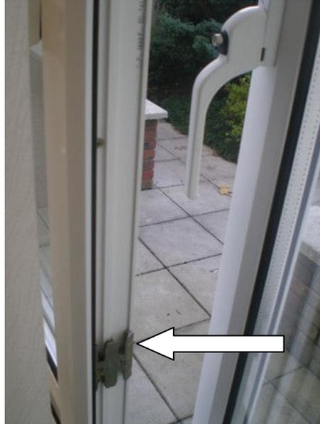
At the bottom of the image above you can see the double latch on the frame of the window. When you have your window fully closed the lock sits in the first latch, on the left in this photo. When you lock the window on the second latch it leaves a gap of over a centimetre as per the following image:
